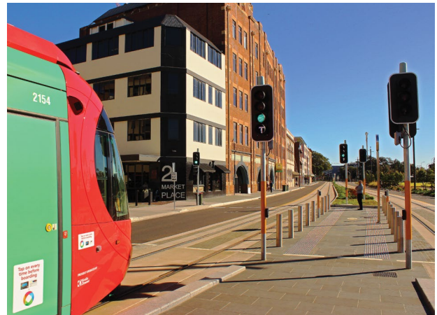
BRAUMS HPSM Central Light Source Traffic Signals on Newcastle Light Rail
